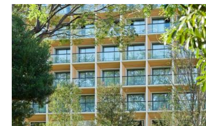
Mitsui Garden Hotel Jingugaien (Improve air conditioning efficiency by adopting balconies that block sunlight)
