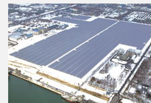
Tomakomai Solar Power Station
