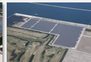
Oita Solar Power Station
