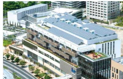
Solar panels on the roof of LaLaport Kashiwanoha
