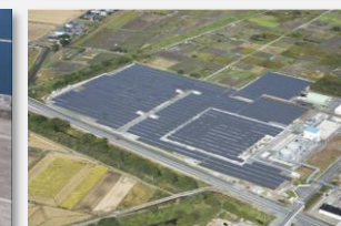
Omuta Solar Power Station
