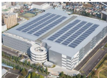
Mitsui Fudosan Logistics Park Hino
