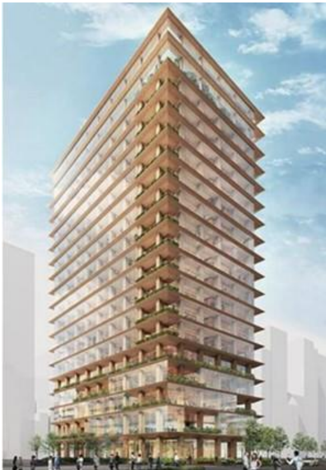
Wooden Office Buildings
