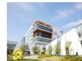
MFLP Funabashi III (Completed in June 2021)
