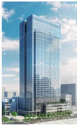
Tokyo Midtown Yaesu (to be completed in Aug. 2022)
