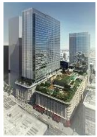
Nihonbashi Takashimaya Mitsui Building (Completed in 2018)
