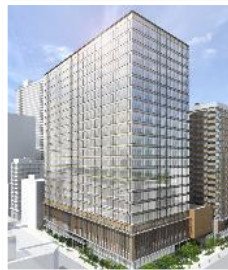
BUNKYO GARDEN GATETOWER (Completed in April 2020)
