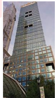
55 Hudson Yards, Inc. (Completed in 2018)
