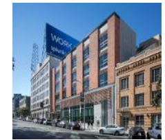
270 Brannan Street (San Francisco)
