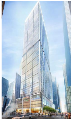
50 Hudson Yards Project
