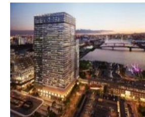
Toyosu 2nd District 2-1 Project
