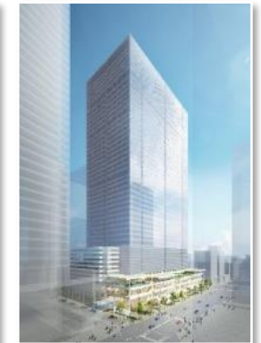
Yaesu 2-Chome Central District (to be completed in FY 2025)
