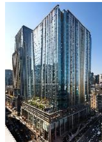
Nihonbashi Muromachi Mitsui Tower
