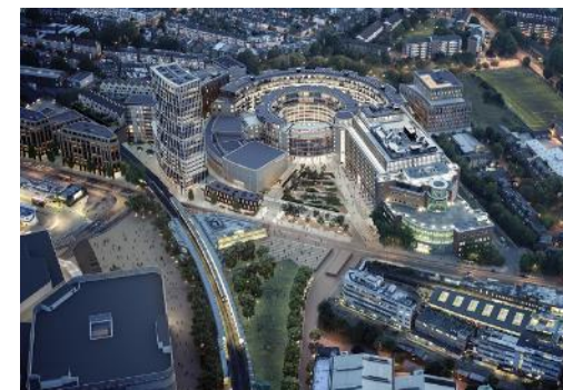
Television Centre Redevelopment Project
