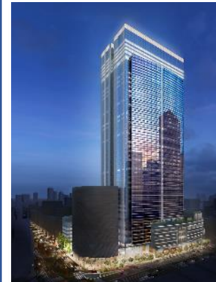
Yaesu 2-chome North District (to be completed in August 2022)
