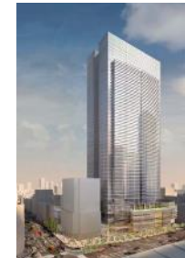
Yaesu 2nd District North Project
