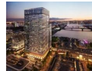
Toyosu 2 nd District 2-1 Project
