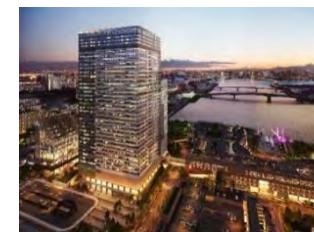
Toyosu 2nd District 2-1 Project
