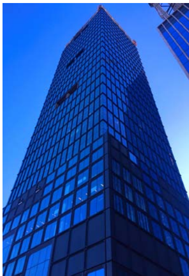
55 Hudson Yards Project
