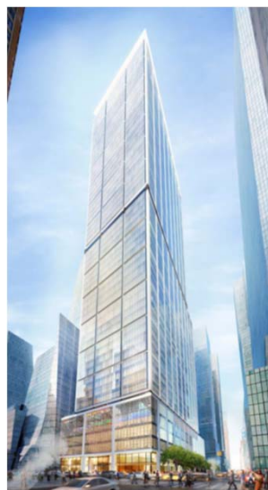
50 Hudson Yards Project
