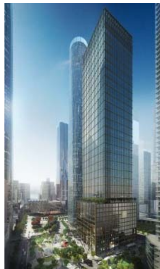
55 Hudson Yards Project
