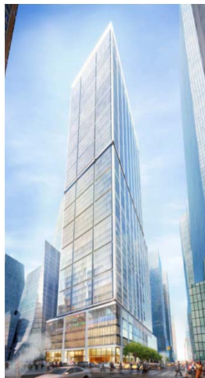
50 Hudson Yards Project
