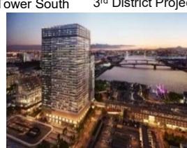
Toyosu 2 nd District 2-1 Project
