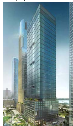
55 Hudson Yards Project
