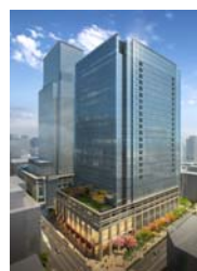
Nihonbashi Muromachi 3 rd District Project
