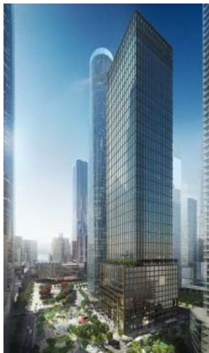
55 Hudson Yards Project
