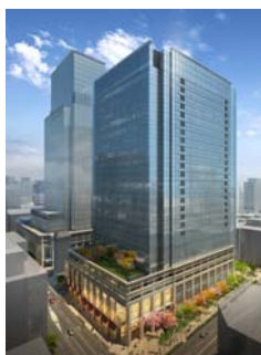
Nihonbashi Muromachi 3rd District Project
