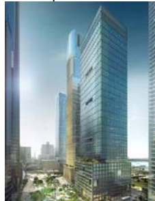
55 Hudson Yards Project
