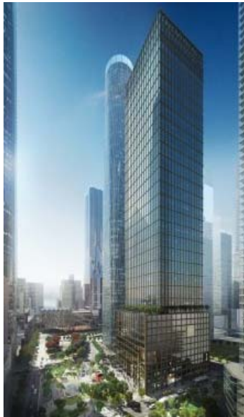
55 Hudson Yards Project
