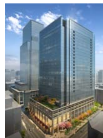
Nihonbashi Muromachi 3 rd District Project
