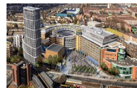
Television Centre Redevelopment Project
