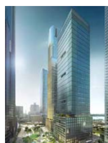
55 Hudson Yards Project
