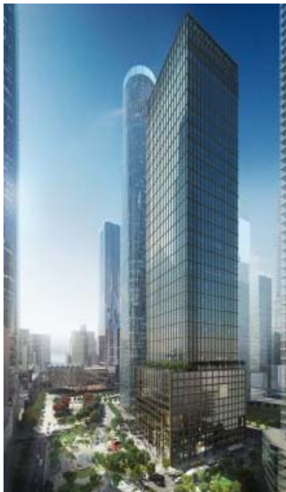
55 Hudson Yards Project
