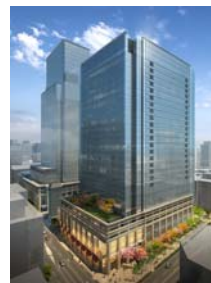
Nihonbashi Muromachi 3 rd District Project
