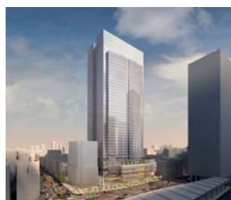
Yaesu 2-chome North Block project
