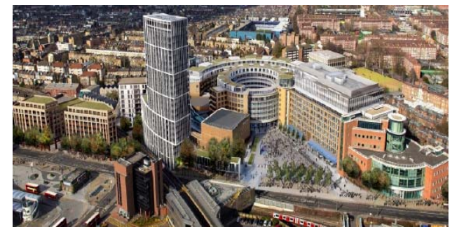
Television Centre Redevelopment Project
