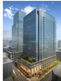
Nihonbashi Muromachi 3rd District Project
