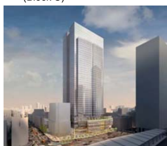
Yaesu 2-chome North Block project
