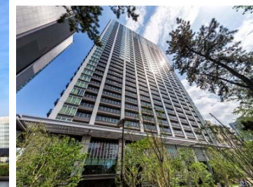
Park Court Chiyoda Fujimi The Tower
