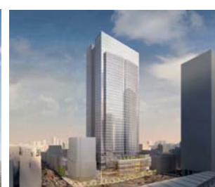
Yaesu 2-chome North Block project
