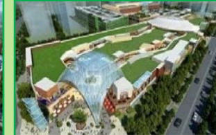
Taiwan Linkou Outlet Project / New Taipei City (2015)
