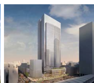
Yaesu 2-chome North Block project
