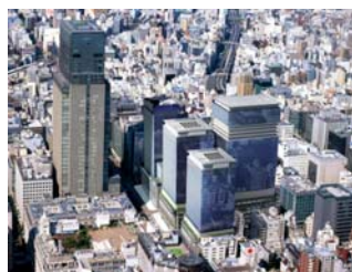
Nihonbashi Muromachi East District Development Project
