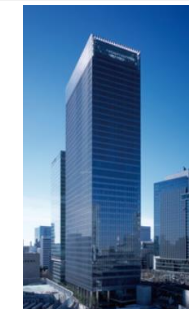
GRAN TOKYO SOUTH TOWER
