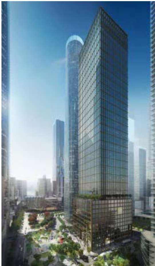
55 Hudson Yards Project
