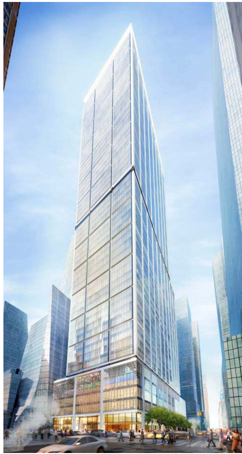
50 Hudson Yards Project
