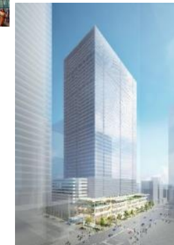
Yaesu 2nd District Central project (scheduled completion FY2025)
