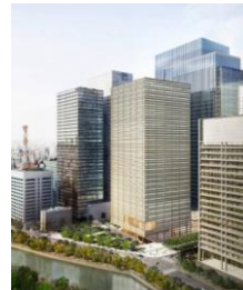
OH-1 Project (scheduled completion February 2020)
