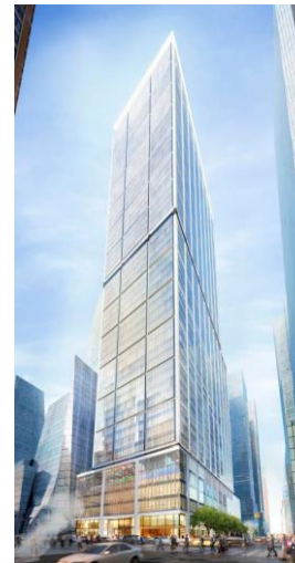
50 Hudson Yards Project (scheduled completion 2022)
