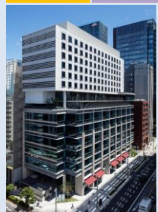
OVOL Nihonbashi Building
