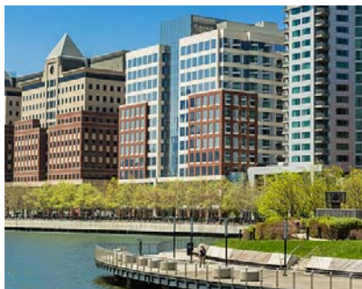
Water Front Corporate Center III
