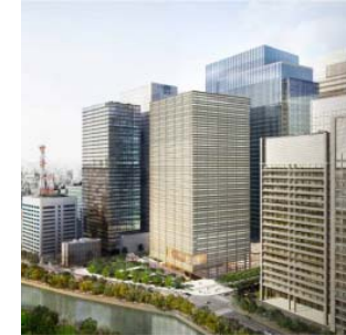
OH-1 Project (FY2019 scheduled)
