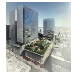
Nihonbashi 2-Chome Urban Redevelopment Project (Block C)
