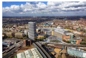
Television Centre Redevelopment Project
