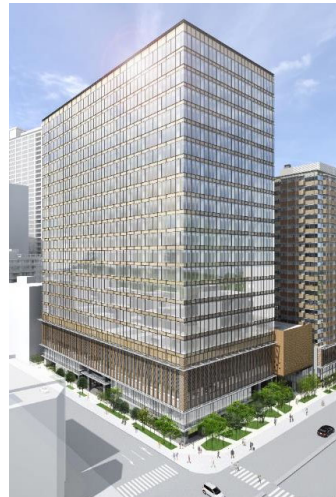
BUNKYO GARDEN GATETOWER (Tokyo, 2020)
