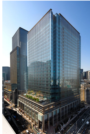
Nihonbashi Muromachi Mitsui Tower (Tokyo, 2019)
