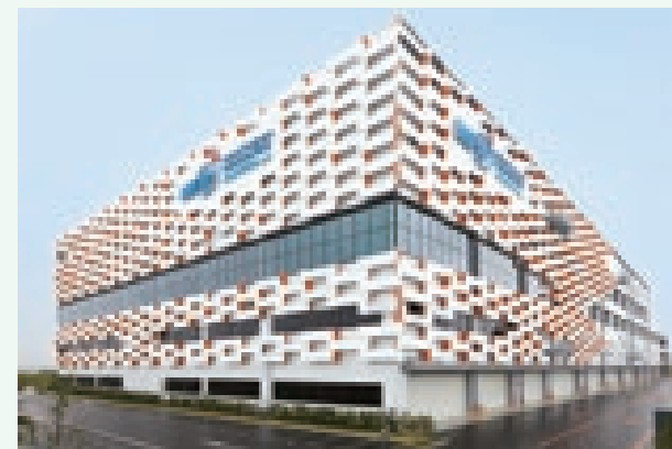
MFIP Haneda (Construction completed in June 2019)
