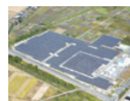
Mitsui Fudosan's Omuta Solar Power Plant
