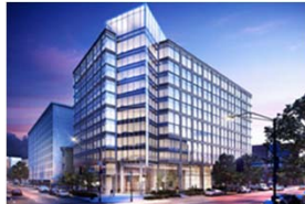
1200 17th Street Project (Washington D.C.)
