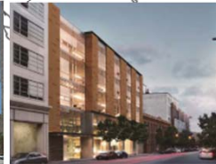
270 Brannan Project (San Francisco)
