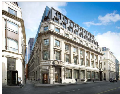
Moorgate Project (UK, to be completed in 2014 Spring)
