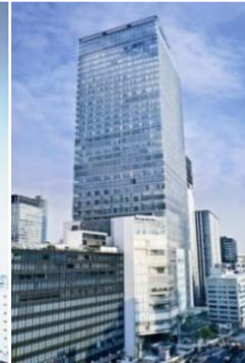
GranTokyo North Tower (2007)
