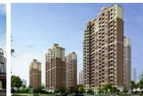
Shanghai New Town Development Project
