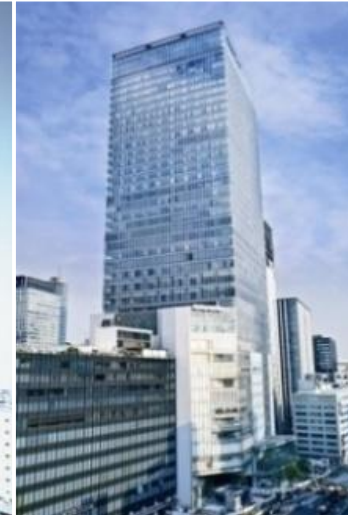
GranTokyo North Tower (2007)
