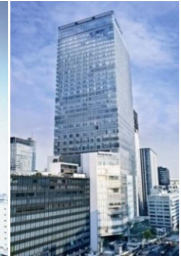
GranTokyo North Tower (2007)
