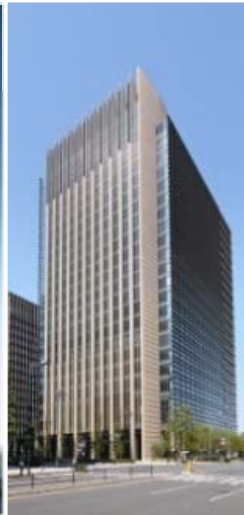
Sumitomo Mitsui Banking Corporation Head Office Building (2010)
