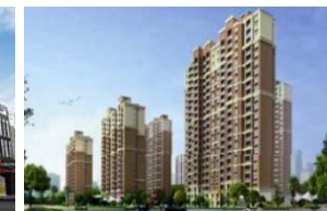
Shanghai New Town Development Project
