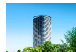
Park Court Akasaka The Tower
