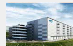
Mitsui Fudosan Logistics Park Ibaraki (MFLP Ibaraki) Ibaraki City, Osaka (completed in September 2017)
