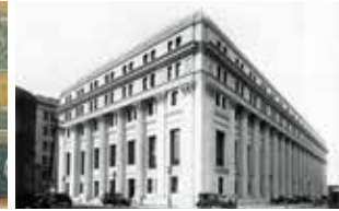
Mitsui Main Building
