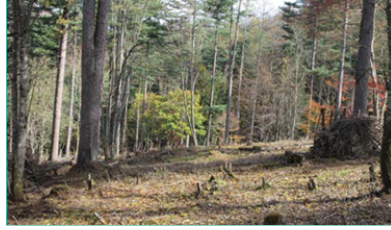
▶ Ground clearing complete
