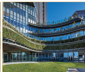
► Wall and roof foliage
