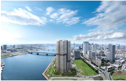
Park Tower Harumi is introducing measures to enhance efficiency
