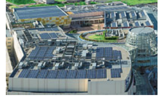
Rooftop solar panels at LaLaport KASHIWANOHA
