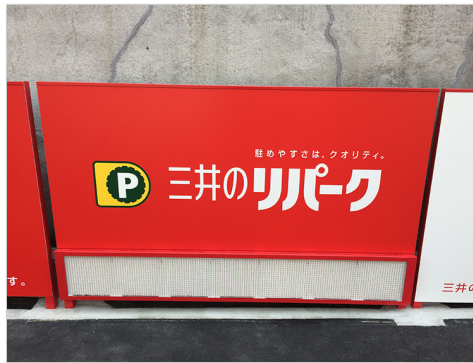
Exhaust gas panel with photocatalytic filter installed at Mitsui Repark's Enkobashi-cho No. 3 Parking Lot in Hiroshima
