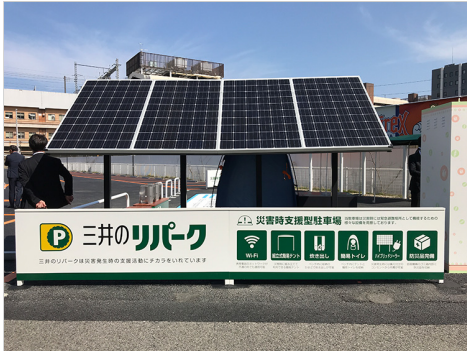
Solar power panels of the hybrid solar system at the Mitsui Repark Minatomachi Niigata Parking Lot
