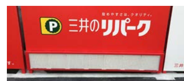
Exhaust gas panel with photocatalytic filter installed at Mitsui Repark's Enkobashi-cho No. 3 Parking Lot in Hiroshima
