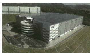
Solar power panels at MFLP Ibaraki (generation capacity approx. 2,000 kW)
