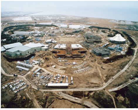
Tokyo Disneyland under construction
