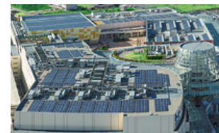
Rooftop solar panels at LaLaport KASHIWANOHA
