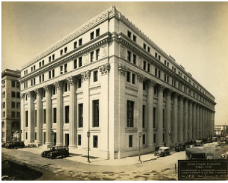
The new Mitsui Main Building (Chuo-ku, Tokyo)
