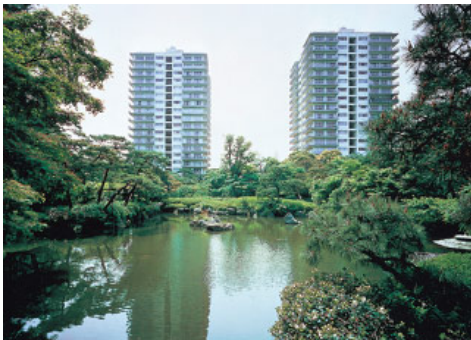
Mita Tsunamachi Park Mansion (Minato-ku, Tokyo)
