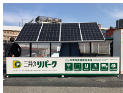
Solar power panels of the hybrid solar system at the Mitsui Repark Minatomachi Niigata Parking Lot
