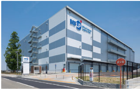
MFLP Inazawa, completed 2017 (Inazawa City, Aichi Prefecture)
