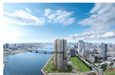
Park Tower Harumi is introducing measures to enhance efficiency
