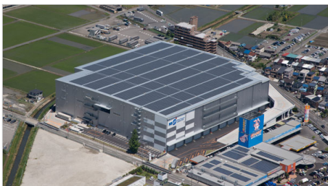
Solar power panels at MFLP Inazawa (generation capacity approx. 1,500 kW)
